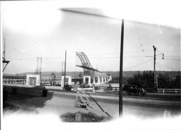
Patullo Bridge Construction Photo from Historical Data Base NW Library
