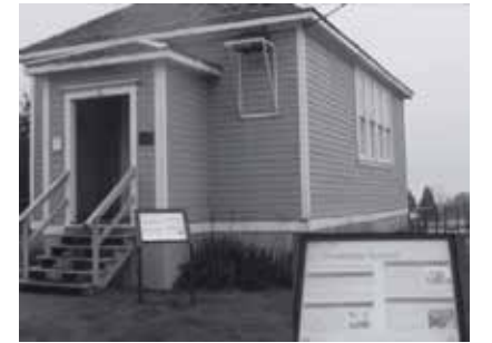
The exterior of the pioneer school as it appeared when used by Surrey students as an operating museum.
