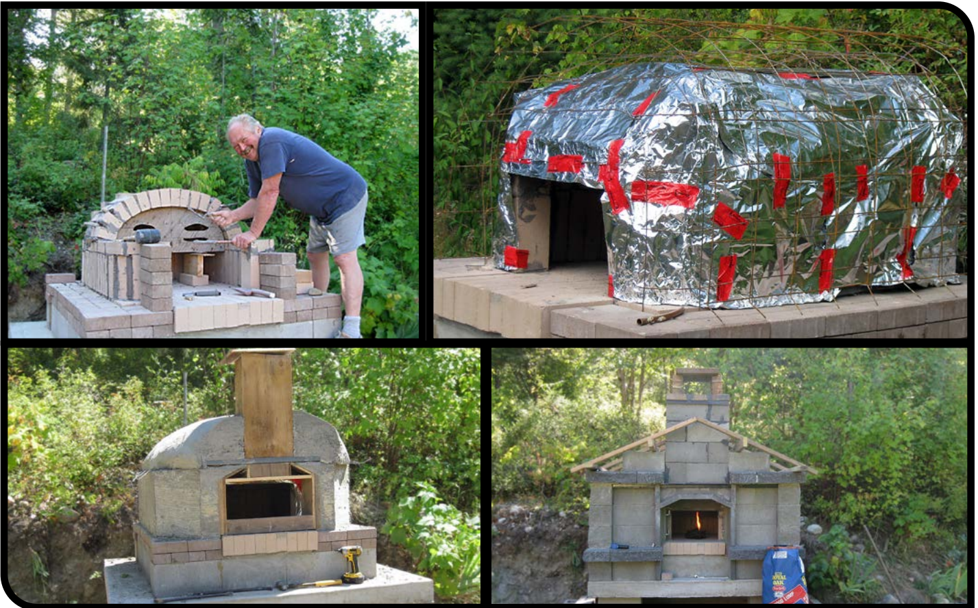
Stages of construction to first fire.
